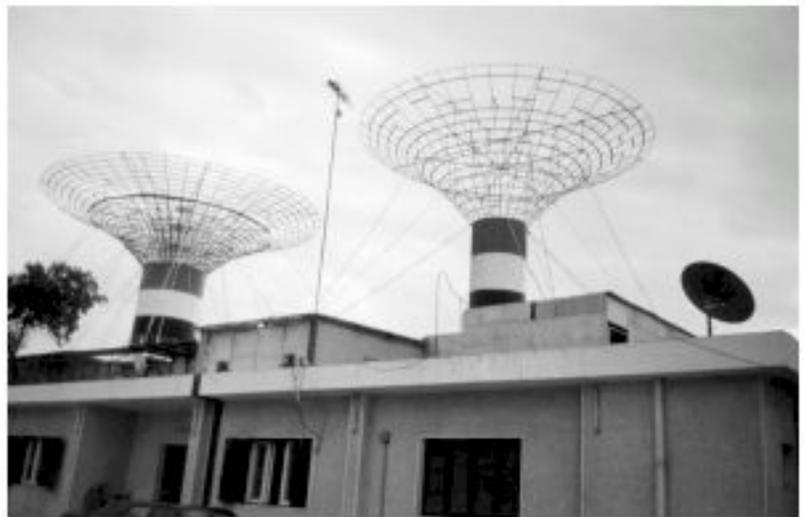
**Fig. 3 The 100kW and 30kW Tanta CFAs situated on the same rooftop, separated by 6m (19.5ft)**
